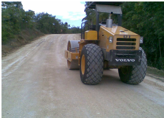
Soil Stabilization of La Paz (Cortes)
