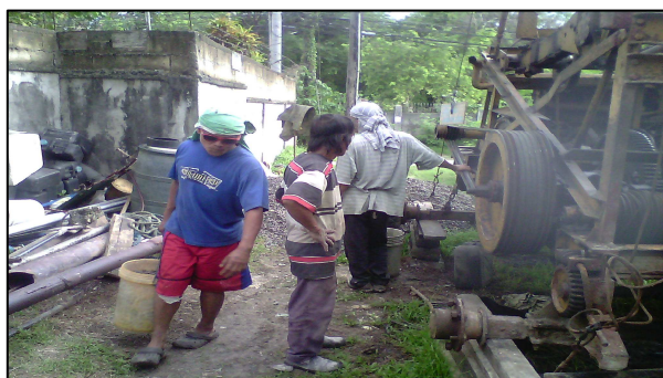
Packing with \frac{3}{4} Gravel on 10" diameter Casing Annular Space
