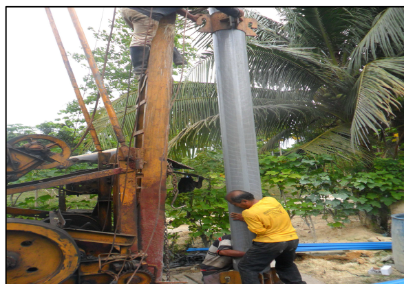
Installation of 10" diameter UPVC Casing
