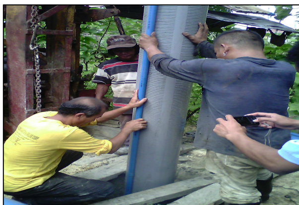
Installation of 10" diameter UPVC Casing
