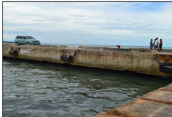
COMPLETED REPLACEMENT OF FENDERING SYSTEM
