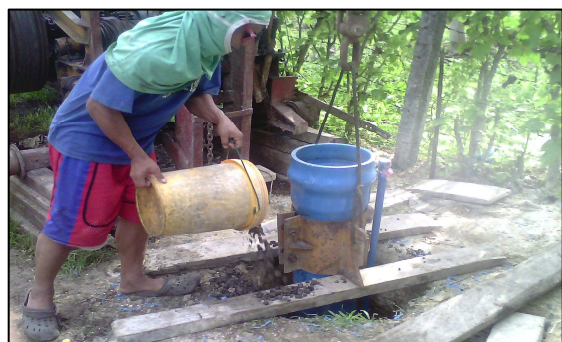
Packing with \frac{3}{4} Gravel on 10" diameter Casing Annular Space
