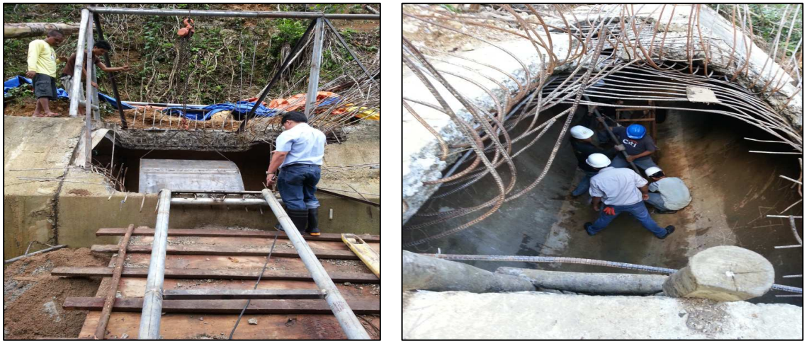
Repair of the JHEP headrace being damaged by the October 15, 2013 earthquake Damaged structures of the JHEP headrace
