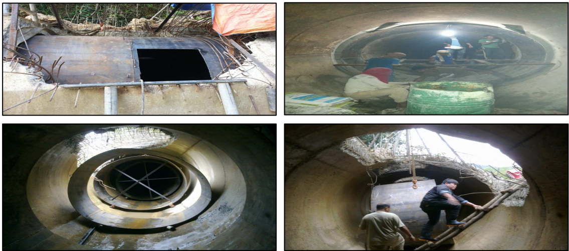
Repair of the JHEP headrace being damaged by the October 15, 2013 earthquake Damaged structures of the JHEP headrace
