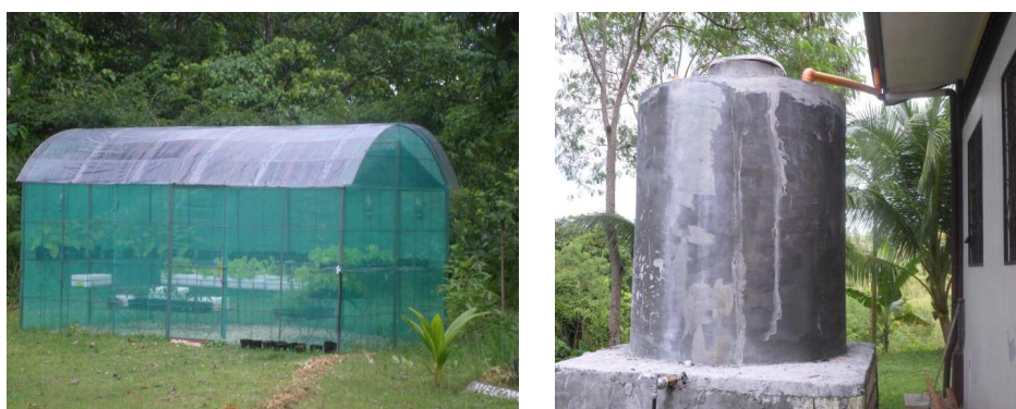
Picture on the right is the showcase mini-greenhouse using hydroponics technology while picture on the left is the showcase 5m 3 cistern using ferro-cement technology to capture and store rain water.
