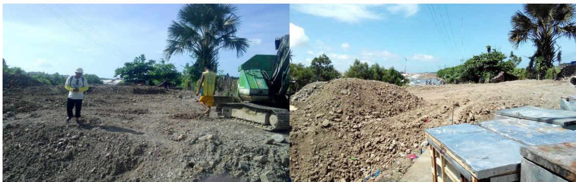
The on-going embankment of the area for the construction of Community Fish Landing Center (CFLC) in Ubay, Bohol
