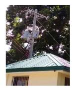
3 Phase Electrical Connection W/ 75 Kva Transformer
