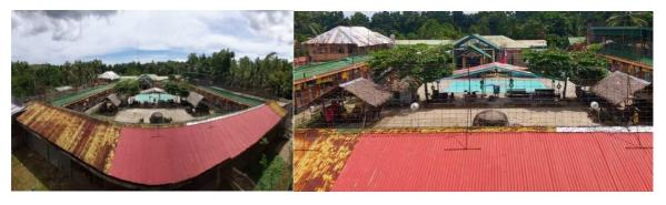
Repainting the corrugated roof from Dorm 12- TC building to prevent further deterioration
