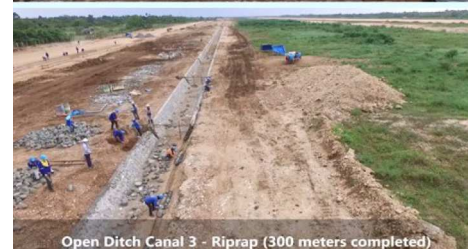
Open Ditch Canal 3 - Riprap (300 meters completed)
