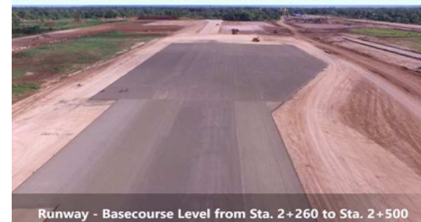
Runway - Basecourse Level from Sta. 2+260 to Sta. 2+500
