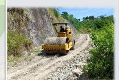
Clearing and Compaction of Access Road
